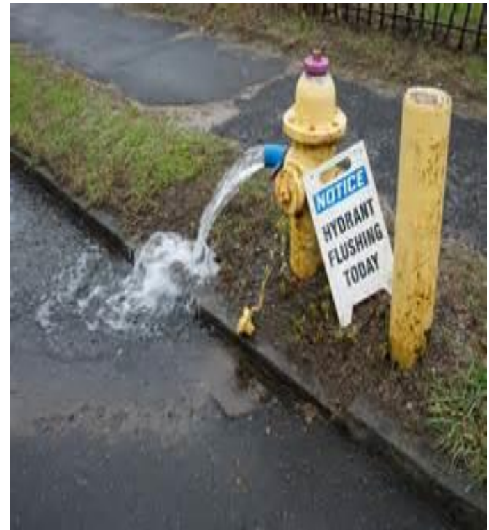
Flushing out discolored water
