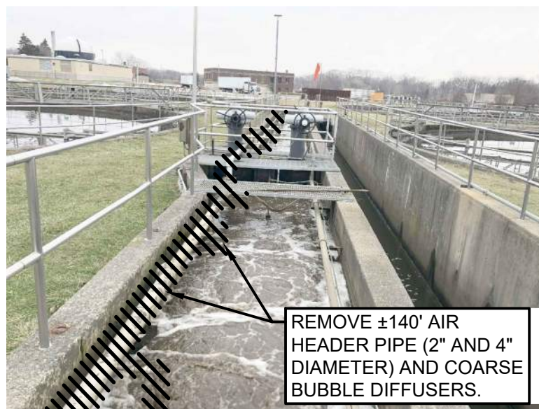
PHOTO 3 - FINAL TANKS 1-4 INFLUENT CHANNEL
