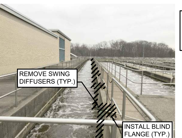
PHOTO 4 - AERATION TANK EFFLUENT CHANNEL
