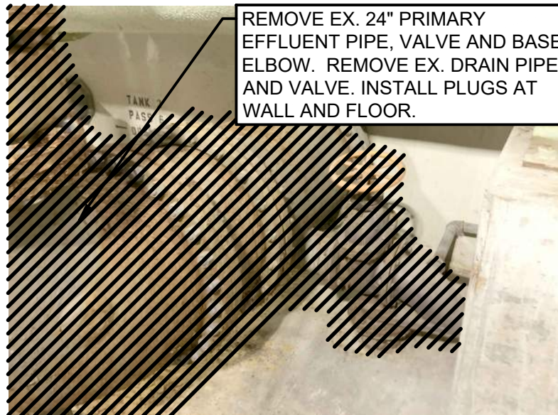
PHOTO 4 - PRIM. EFF. AND DRAIN PIPE
