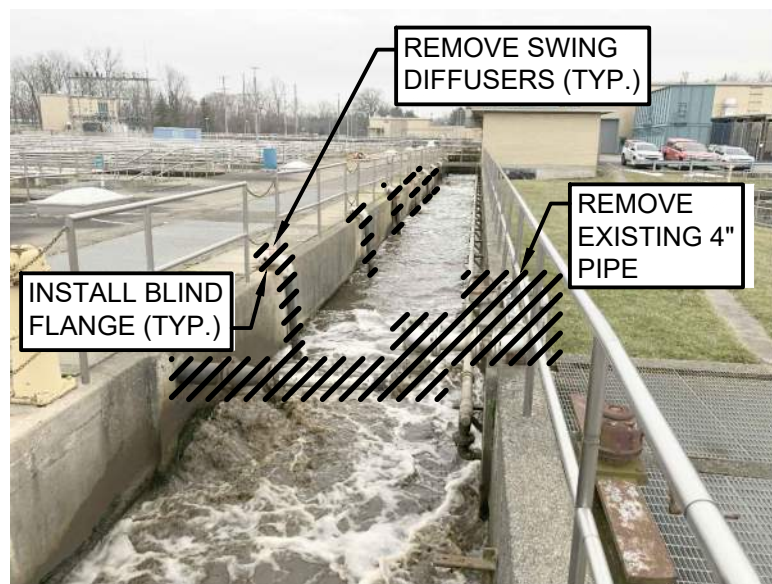
PHOTO 1 - AERATION TANK EFFLUENT CHANNEL
