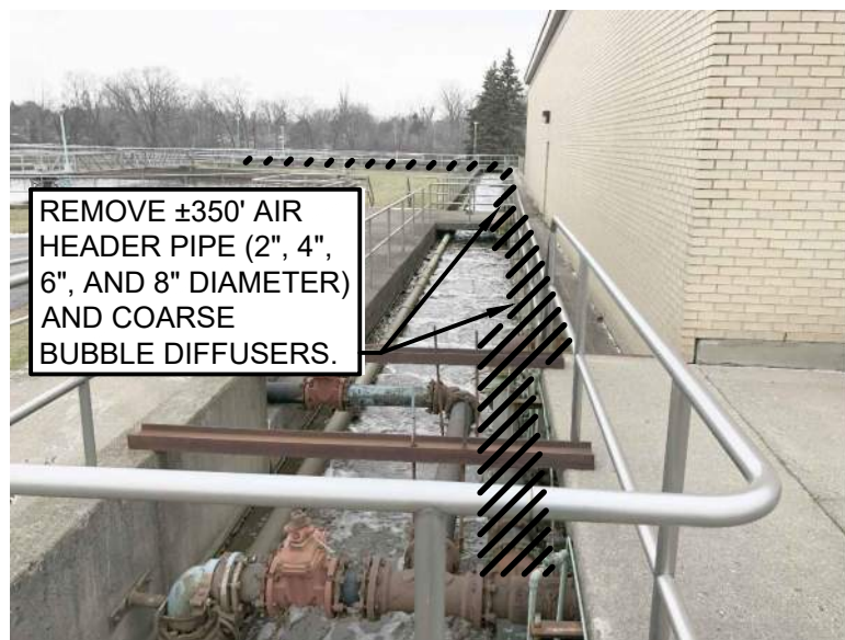
PHOTO 2 - FINAL TANKS 5-8 INFLUENT CHANNEL
