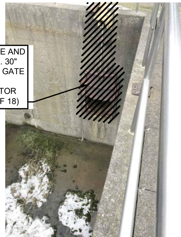
PHOTO 1 - STEP FEED SLUICE GATE
