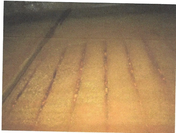
Corrosion of Vertical Wall Reinforcing
