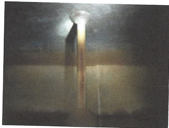
Column Deterioration and Corrosion
