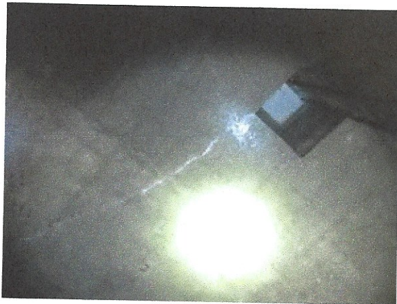
Roof Slab Crack at Re-Entrant Corner
