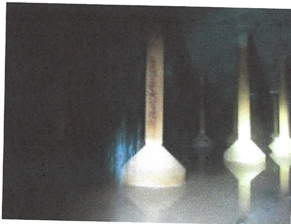
Column Deterioration and Corrosion, with Active Roof Leak at Expansion Joint
