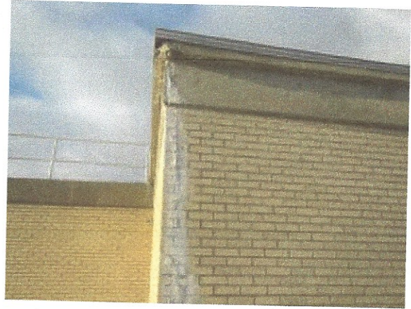
Inlet Structure Exterior Wall Cracking
