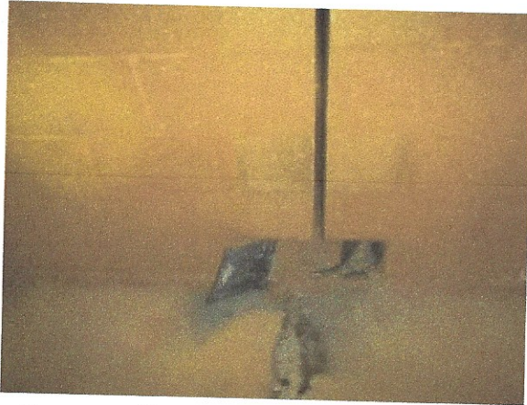
Masonry Baffle Wall Joint Filler Displacement
