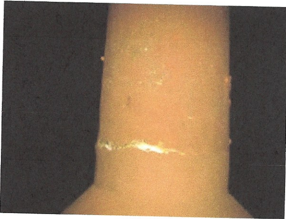
Circumferential Crack and Bulging near Column Pedestal
