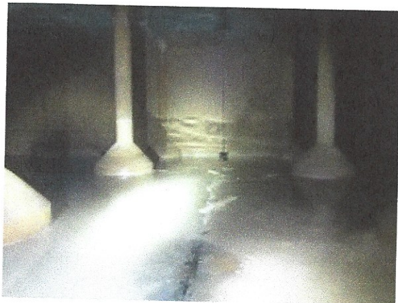
Deteriorated Premolded Joint Filler at Type E3 Expansion Joint
