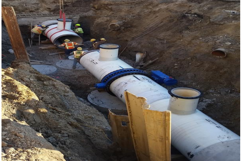
KWA pipeline construction
