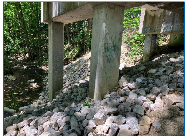
April 2023- Trestle T-2 looking West after backfill and rip rap placement
