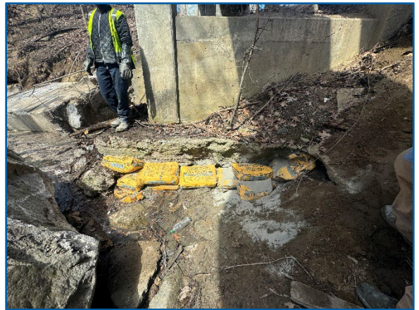
April 2023- Trestle T-2 after grout bags and debris removal
