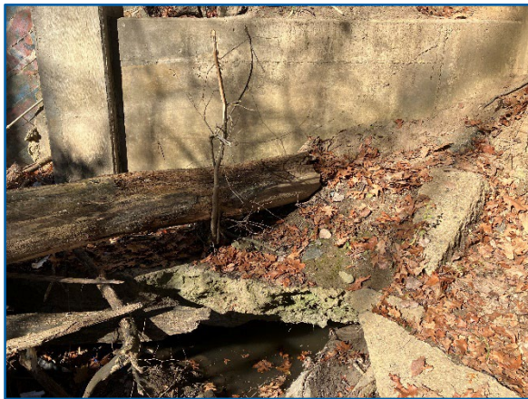
November 2023- Trestle T-2 before grout bags and debris removal
