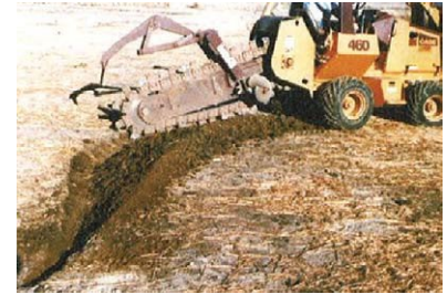
Figure 15. Trenchers make a wider excavation at turns.
