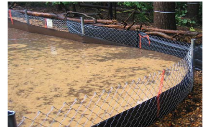
Figure 11. Chain link supported silt fence
