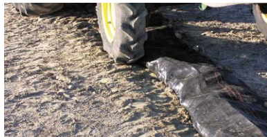
Figure 13. Tractor wheel compacting the soil
