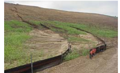
Figure 23. New silt fence below the old fence
