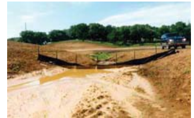
Figure 8. Proper installation, bottom of both ends are above the top of the middle.
