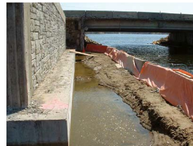
Figure 19. Silt fence for bridge abutment excavation.
