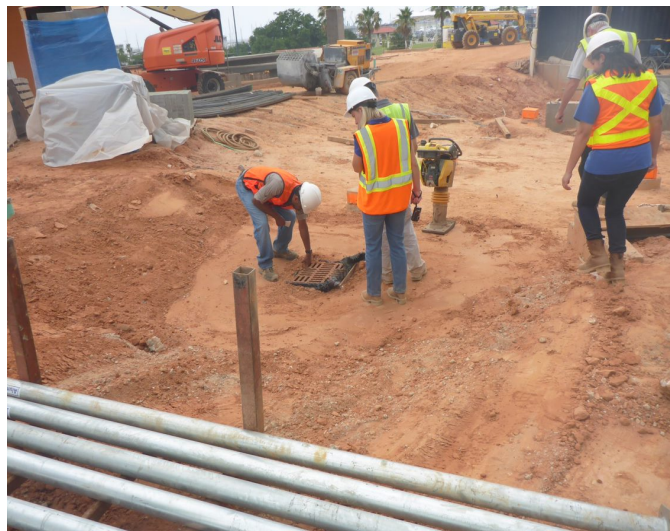
Construction staff inspecting a storm drain with inlet protection in an active construction area.
