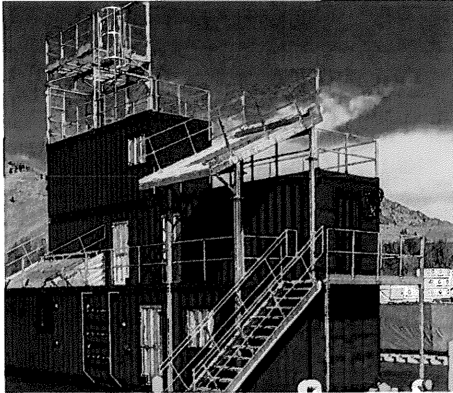
Example Training Tower Structure Image
