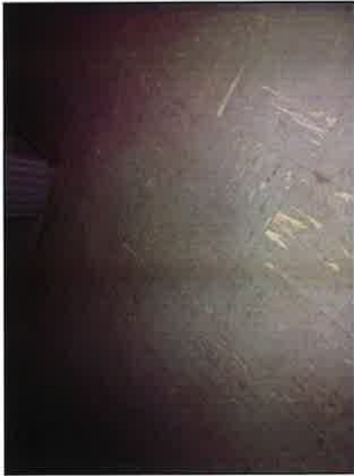
9" Gray Floor Tile with Tan Streaks and Mastic
