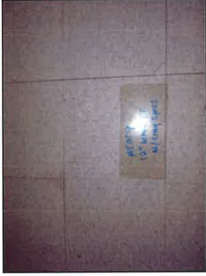
MM9 12" White Floor Tile with Gray Streaks and Mastic
