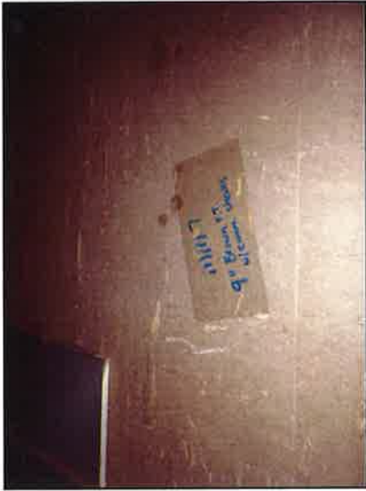
MM7 9" Brown Floor Tile with Cream Streaks and Mastic
