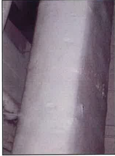
TSI4 Canvas Wrap over Fiberglass Duct Work
