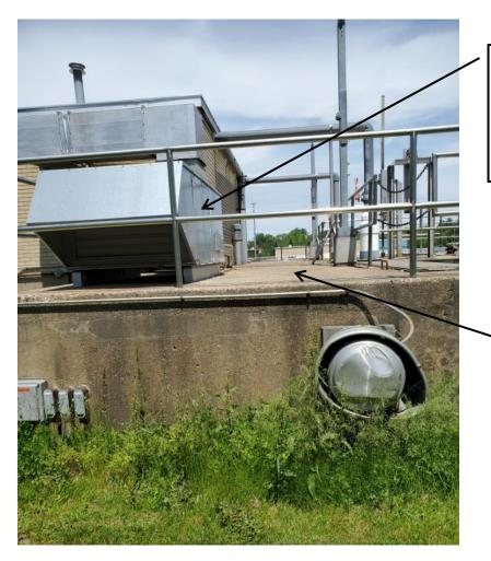
Existing HVAC to be temporarily removed, then replaced once existing venturi meter has been replaced with proposed magnetic meter for Battery A Grit.
